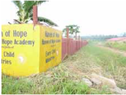
Security fence, completed this year
