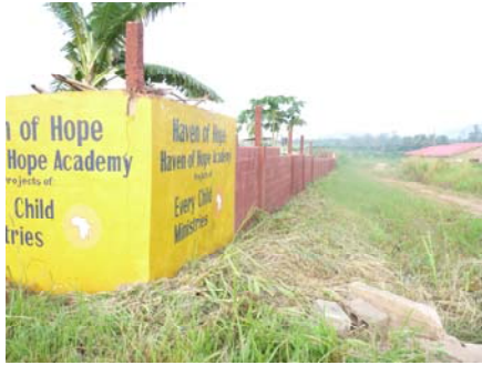
Security fence, completed this year
